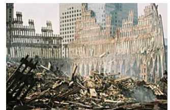
The exterior support columns from the lower level of the South Tower remained standing after the building collapsed.
